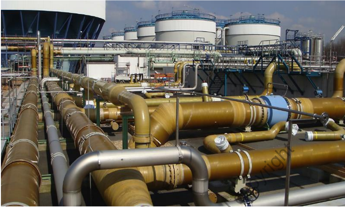
Figure 2.1. Use of GRE composite pipes in the oil and gas industries (EMCO, 2015).
