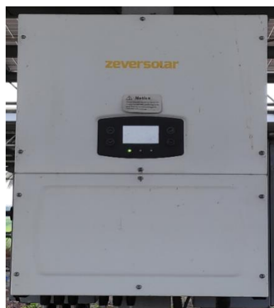
Figure 2. Zeverlution Pro 33K DC to AC inverter
