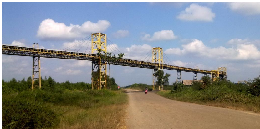
Figure 2.4: Example of Coal Conveyor in Indonesia (Joppe, 2011)
